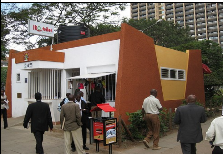
Ecotact, one of the companies The Acumen Fund has invested in, builds and operates these pay-per-use toilets.
